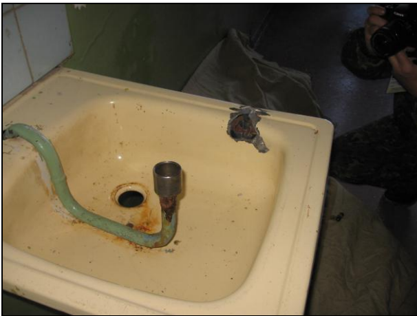
Shrapnel from a shell broke a sink in the school bathroom. There is no possibility of reglazing the windows, so they were covered with cardboard
